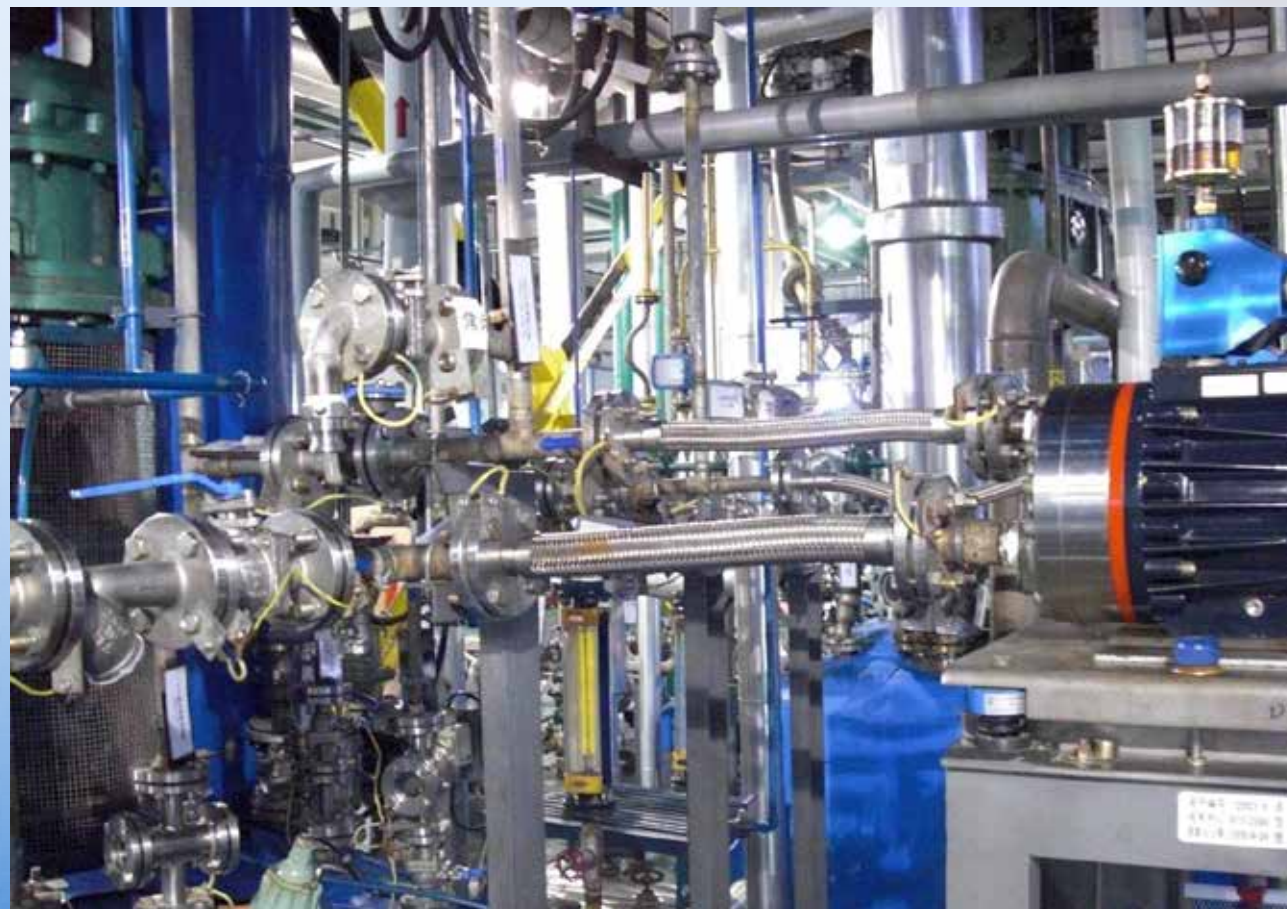
Injection of proprietary monomers and inhibitors
